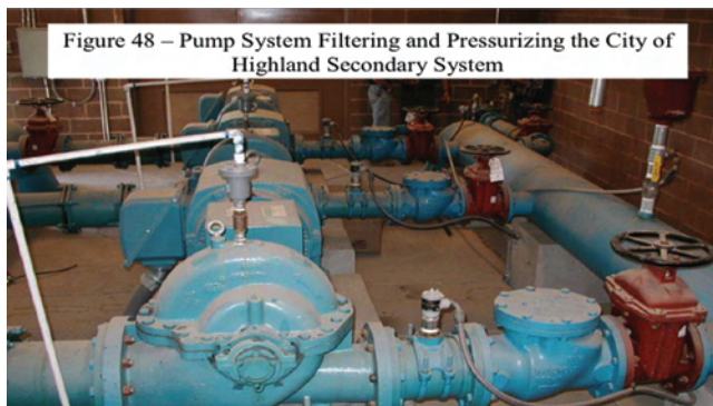
Figure 48 – A pump system filters and pressurizes Highland's system.
