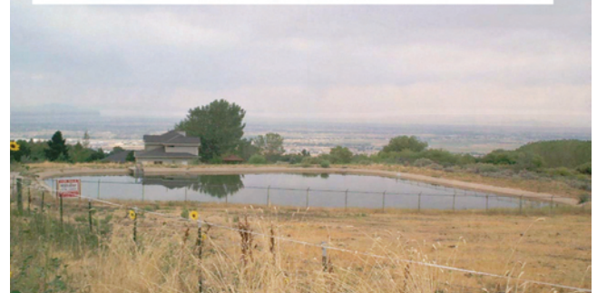
Figure 41 – Small Storage Facility that Pressurizes Secondary Water Delivery in the North Ogden Area, under the Pine View Water Users Association
