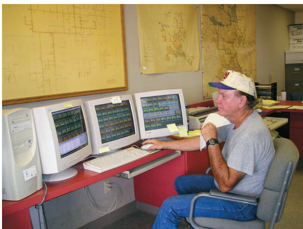
Figure 4. An operator at the Central Arizona Irrigation and Drainage District near Phoenix monitors primary flows and water surface elevations on the 60-mile canal. The SCADA system was implemented at relatively low cost using affordable RTU equipment and spread spectrum radios for communication.
