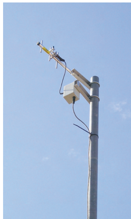
Figure 5 shows a spread spectrum radio and a directional antenna installed on a galvanized steel pipe at one of CAIDD's check structure sites.
