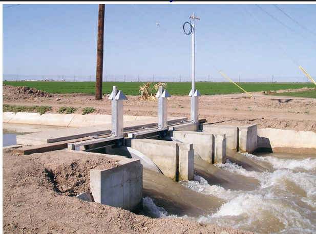
Figure 3. This check structure is controlled by Rubicon gates integrated with the SCADA system and used for water surface level control or flow control.
