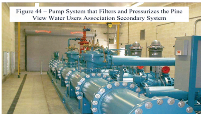
Figure 44 – The pump system filters and pressurizes the Pine View Water Users Association Secondary System.
